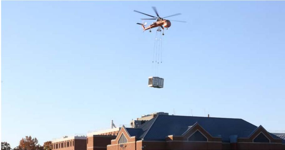
*An air-crane was used to remove the older, failed cooling tower equipment off of the main hospital, building 200, and to install the new, energy efficient cooling tower equipment onto the roof.*
