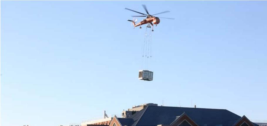
*An air-crane was used to remove the older, failed cooling tower equipment off of the main hospital, building 200, and to install the new, energy efficient cooling tower equipment onto the roof.*
